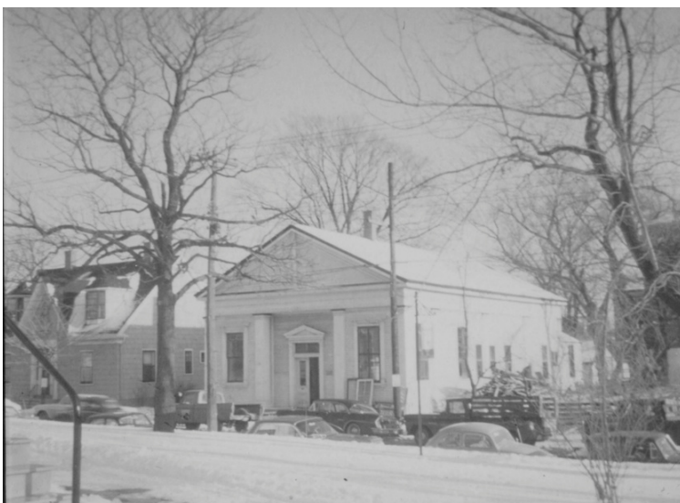
The Mechanics Institute, designed by Henry Elliot DHM 1993.015.1144
